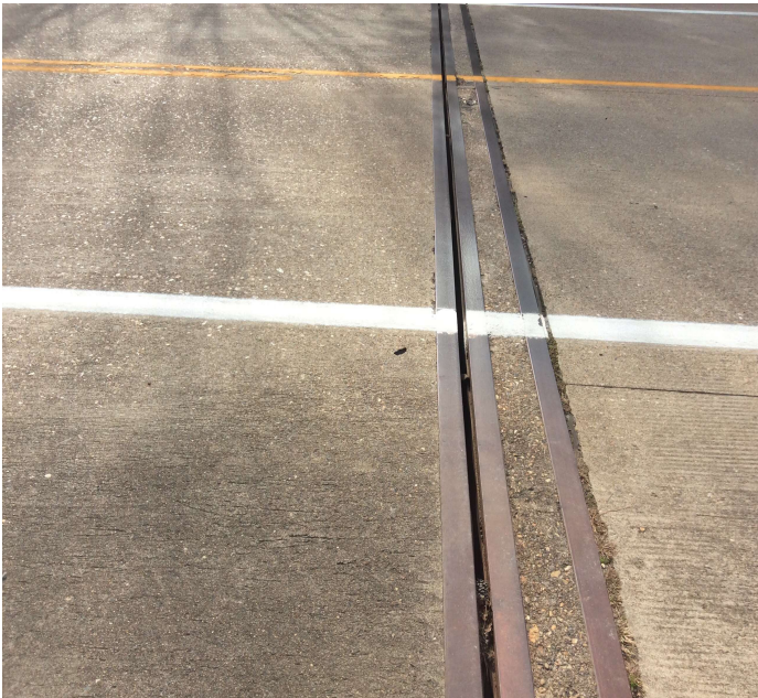
PHOTO 1 Description Bent 1 joint seal missing
